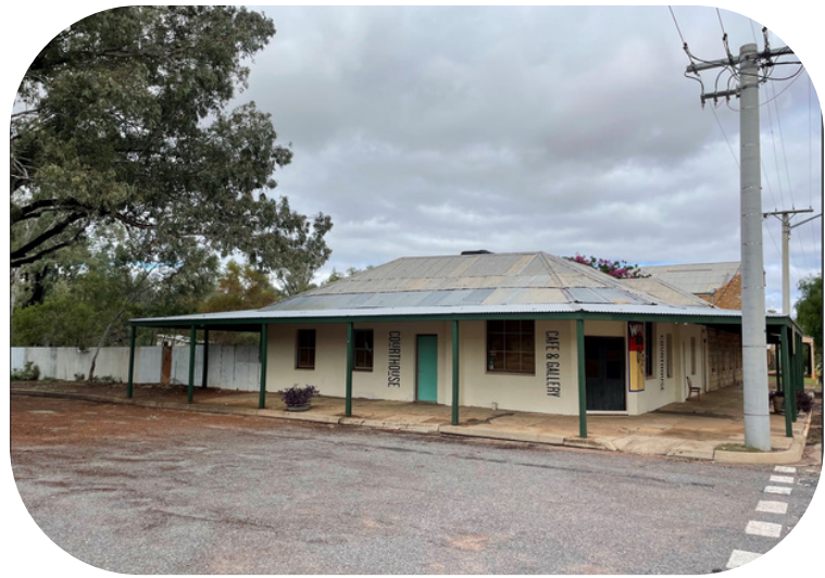
Street view of Wilcannia Community Hub Property
